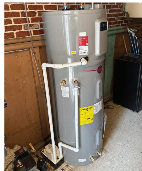
Heat Pump Water Heater
