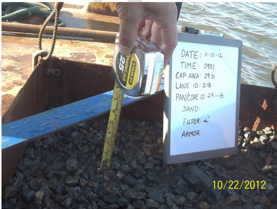
Photo 2: Filter thickness verification in Cap Area 29B.
