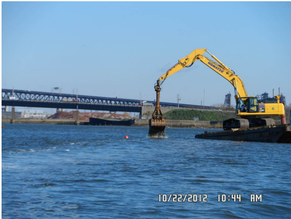
Photo 1: Mechanical placement of armor in Cap Area 17.
