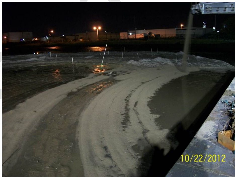
Photo 4: Placement of sand using Telebelt in Cap Areas 6 and 13.
