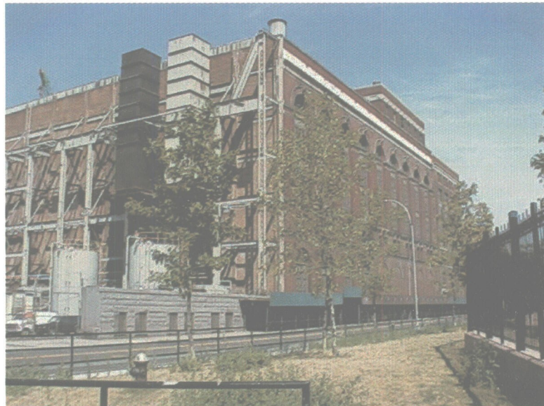
Southern exposure of Kent Avenue Station.
