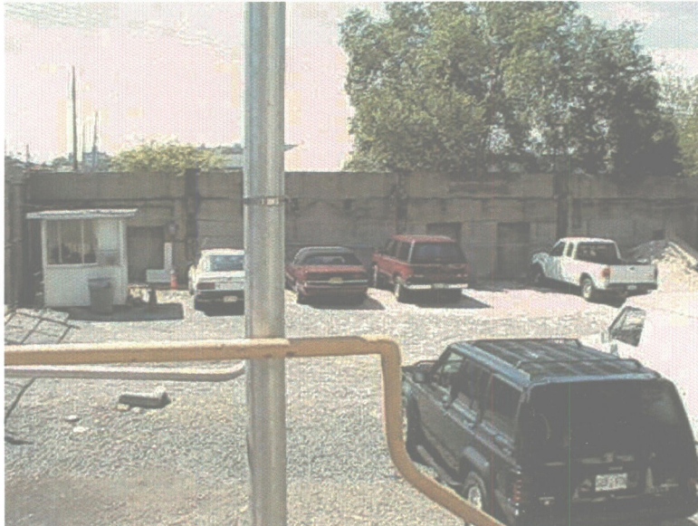
Remnants of south wall of the former Williamsburgh Boiler House.
