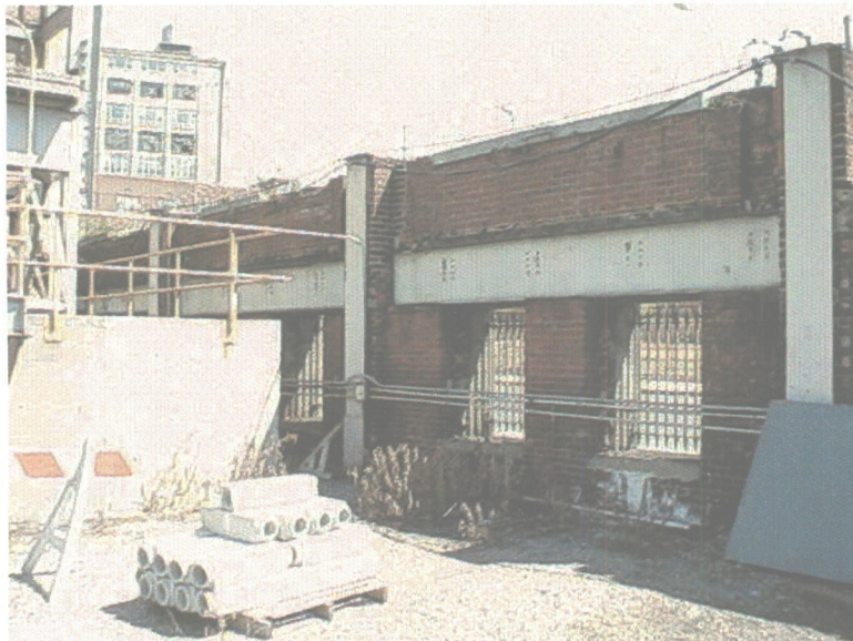
Remnants of east wall of the former Williamsburgh Boiler House.
