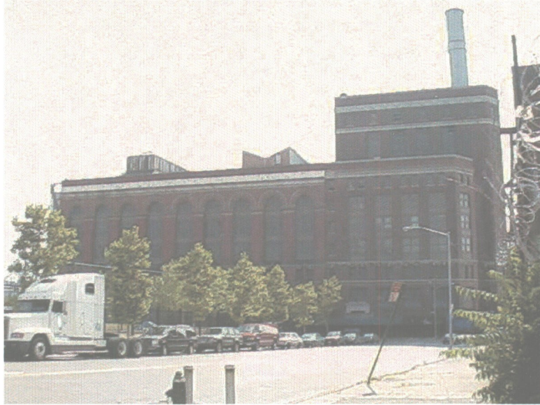
Eastern exposure of Kent Avenue Station
