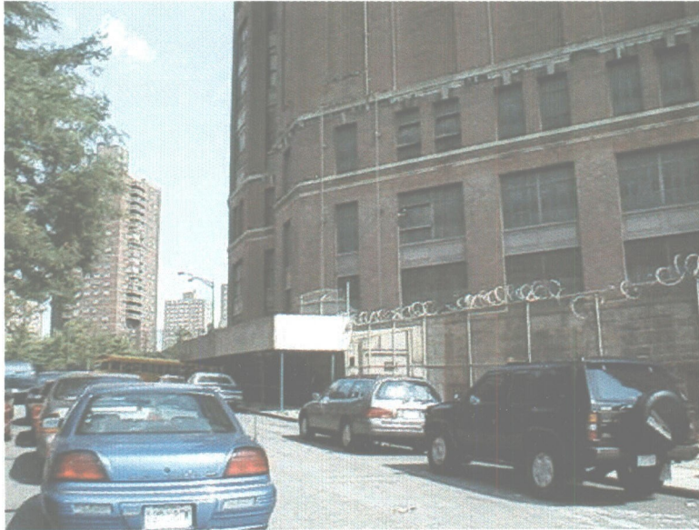
Northern exposure of Kent Avenue Station.
