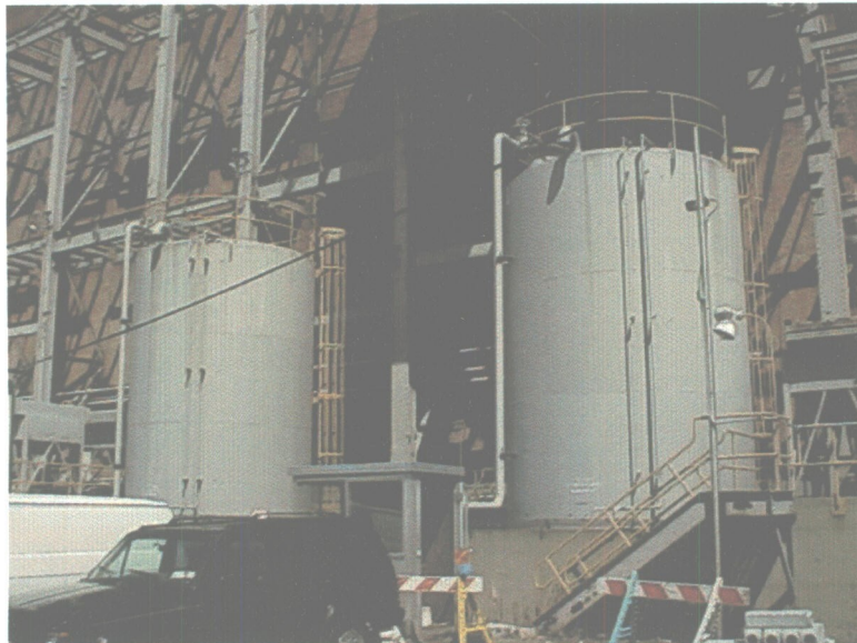
Former 40,000-gallon kerosene storage tanks and steel structural members from former Williamsburgh Boiler House.
