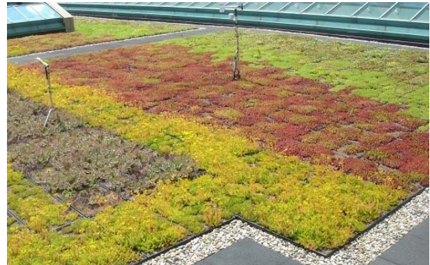
Figure 1: Photograph of the green roof modular system after one year showing above-grade monitoring stands
