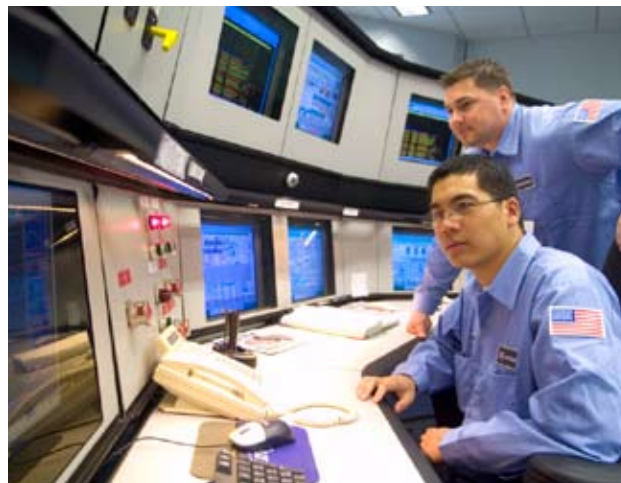
Con Edison uses the latest available technologies to monitor system performance.
