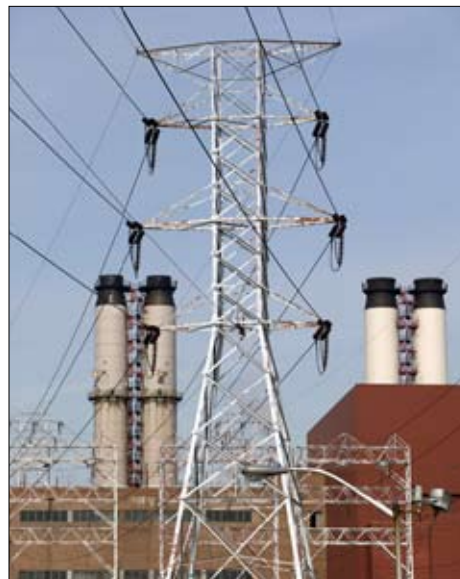
Con Edison's transmission system takes electricity from power producers.
